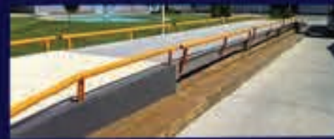
Installation with access ramps
